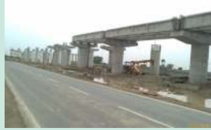
Project: Flyover • Location: Jhajjar Riwari Road (Haryana) • Client: Railway • Status: Inprogress
