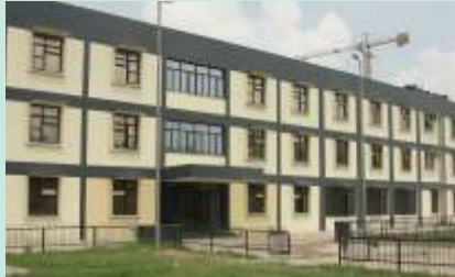
Project: Railway Gaurd's & Driver's Rest House • Location: Opp. Tughlaqabad Metro Station • Client: Railway • Status: Completed
