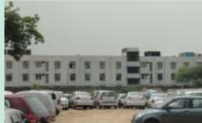
Project: Running Room • Location: Tughlaqabad • Client: Railway • Status: Completed
