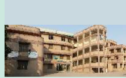
Project: School • Location: Loni Road, Shadhara • Client: PWD • Status: Completed
