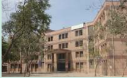
Project: School Building • Location: Dilshad Gardan • Client: PWD • Status: Completed
